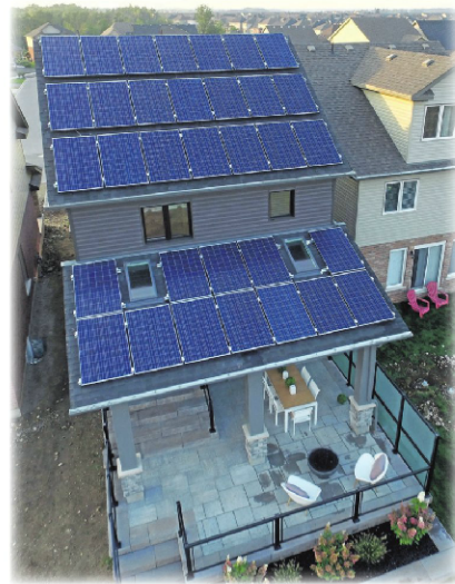
A 'discovery home' is now open for viewing and is generating power from a 33-panel photovoltaic rooftop system.
