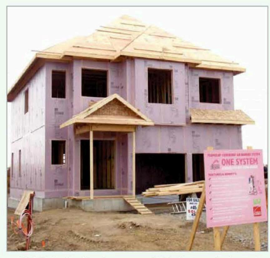
"Affordability is achieved through conservation first before generation," says Ciarlo, noting that the key components of a NZE home are: outstanding insulation, a tight building envelope with high-performance windows and, right-sized efficient mechanical systems for heating and cooling.
